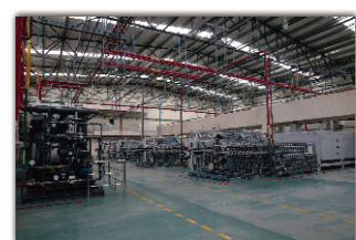
制粉车间 Powder Process Workshop
